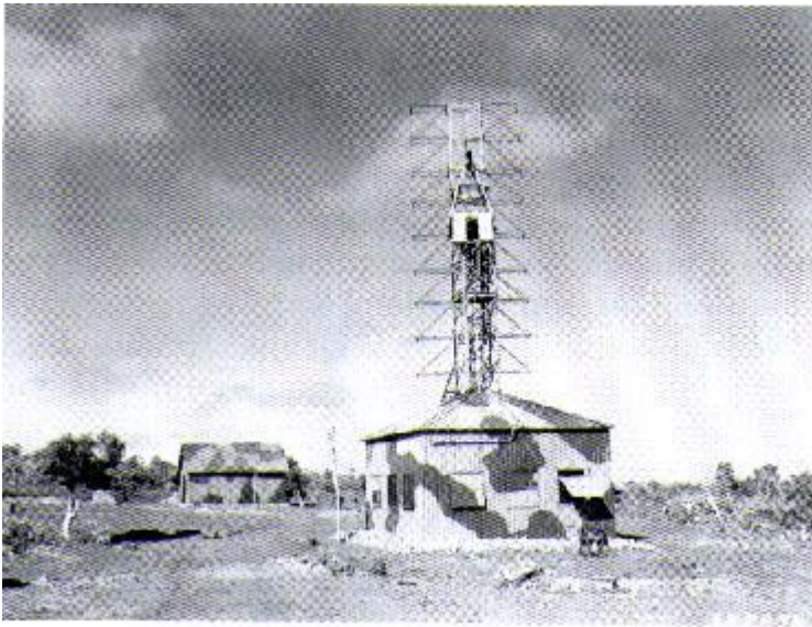
SCR-271 3 m air warning radar at New Caledonia in May 1943. The SCR-271 was an early version of the SRC-270.
